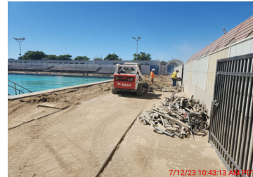
Demolition of Existing Deck
