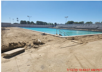
Demolition of Existing Deck
