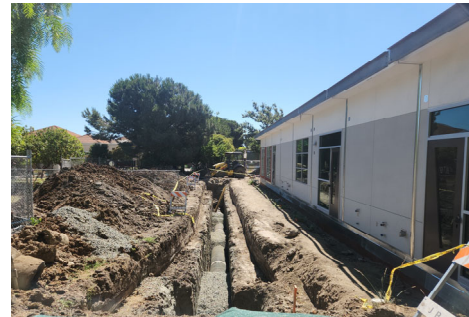
Project Site - Installation of Underground Utilities
