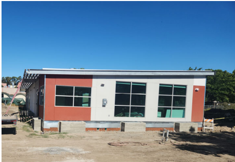
Modular Building Installed on Foundation System
