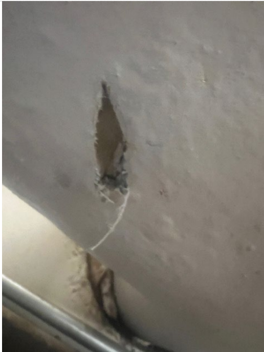
Gray Pipe Wrap with Fiberglass – 3% Chrysotile
