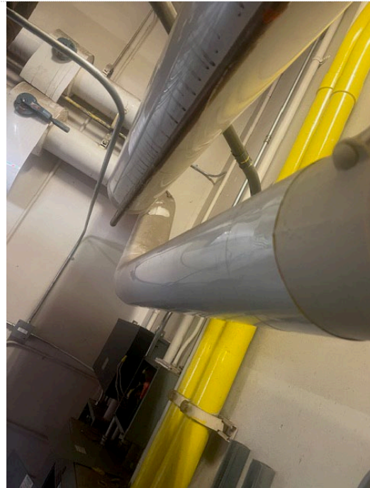
Yellow Pipes are Lead-Containing
