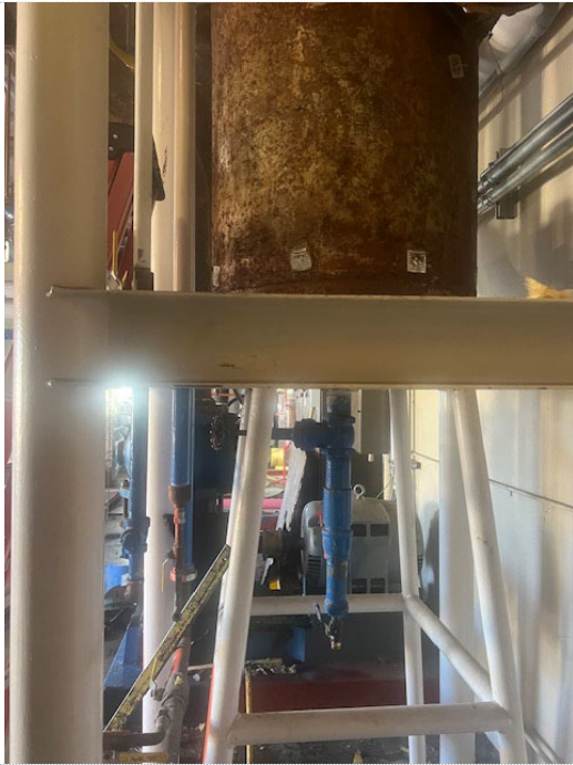
White Paint on Steel Lead-Containing
