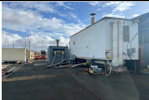
Temporary Boiler Installation
