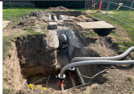
Emergency Underground Hydronic Piping Repairs
