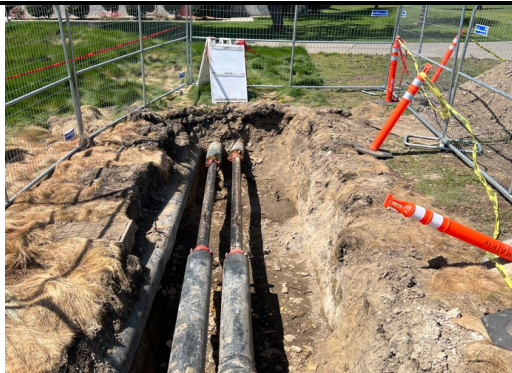
Emergency Underground Hydronic Piping Repairs
